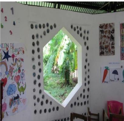
The classroom is constructed using plastic bottles and earth-bag technology. The earth bags are used as structural columns for the roof, and the bottles are used to fill in between the earth bag columns.
